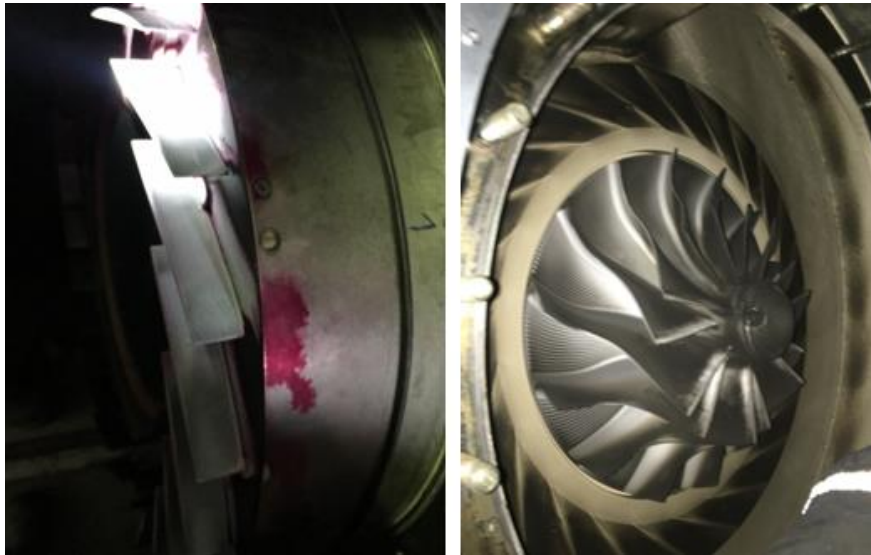
Figure 3: Penetration test and impeller check in a preventive maintenance
